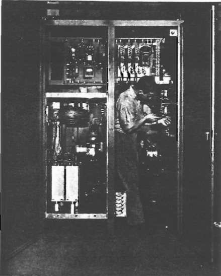
FIG. 5-3B. Interior view of a water-cooled 25-kw 450-kc generator showing the oscillator on the left and the power supply on the right. (General Electric Corp.)
