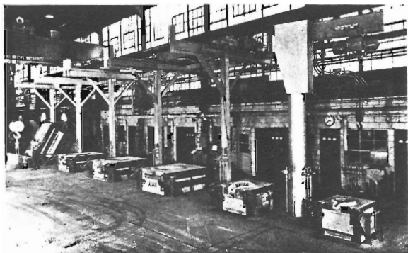
FIG. 3-37. A large-scale steel-melting induction-furnace installation. ( Sandusky Foundry and Machine Co. )
