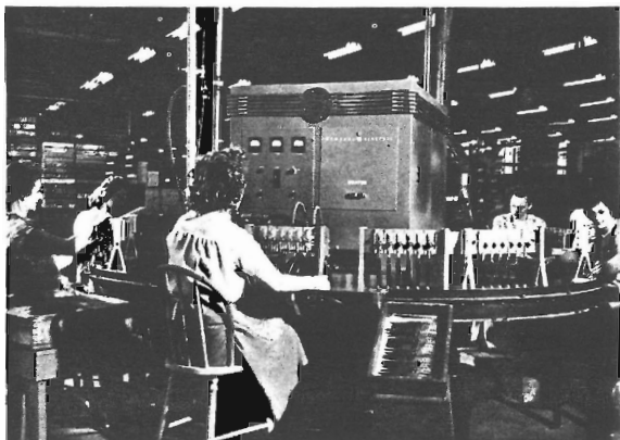
FIG. 3-20. Batch production of knife-handle brazing at a r-f power of 530 kc. ( Oneida Ltd. )
